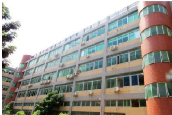
Factory Building Hall
