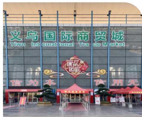
Commercial Centre: KVD188D
