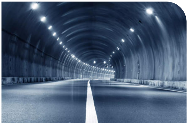
Tunnel in Madrid, Spain:KVD188D
