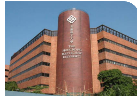
HK University Project renovation: KVD188D
