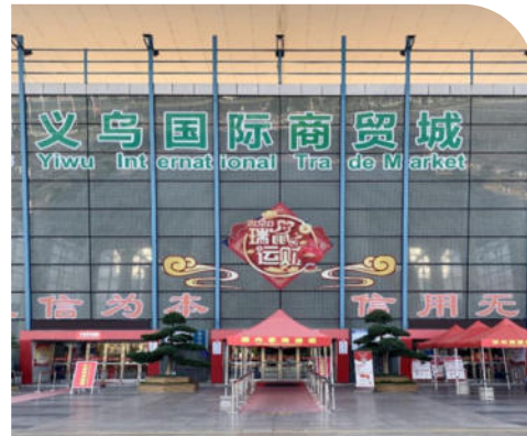
Commercial Centre: KVD188D
